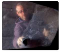
On the grid If you work a section of the window at a time on both sides, you can see how many bits you've missed. Apply in a rotary motion, and keep dabbing on more polish. As you rub, you'll feel the cloth start to drag.
